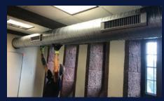
Air exchange units are being installed in quad classrooms to increase fresh air flow.
